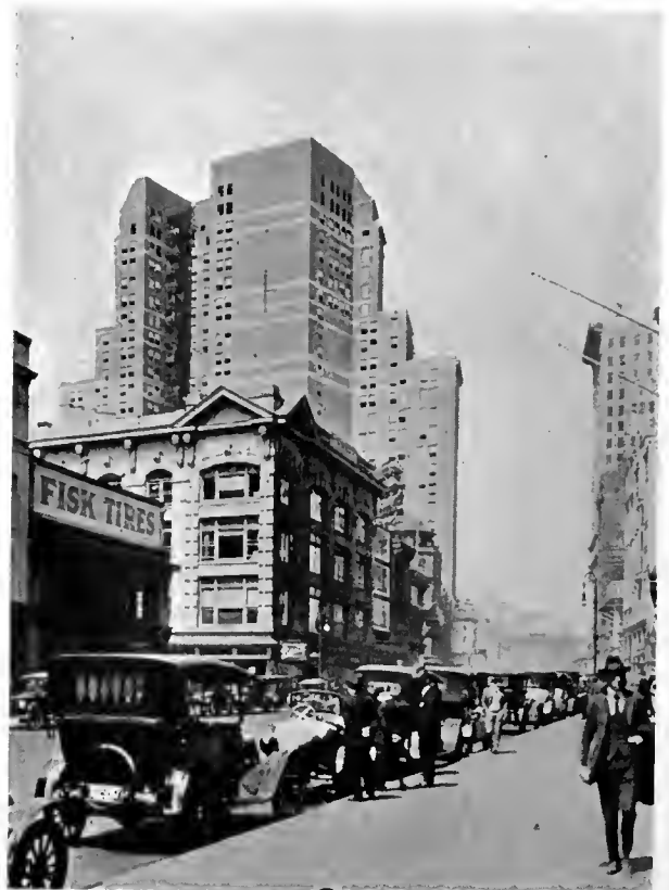
FIG. 4. REAR VIEW OF FISK BUILDING, BROADWAY AND 57th STREET, NEW YORK
